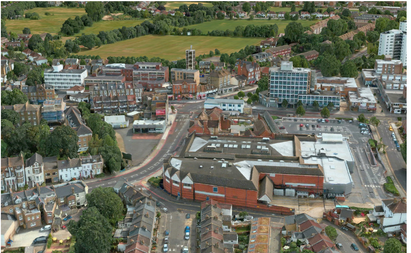
Figure 1: Aerial view of Lee's District Centre (Source: BU1-Session 1- 11 January 2018)
