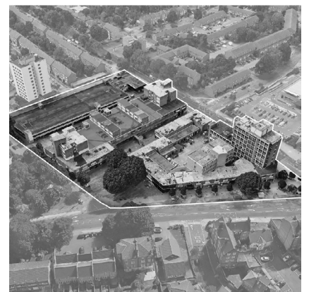
Figure 09 Ensemble of Leegate complex
