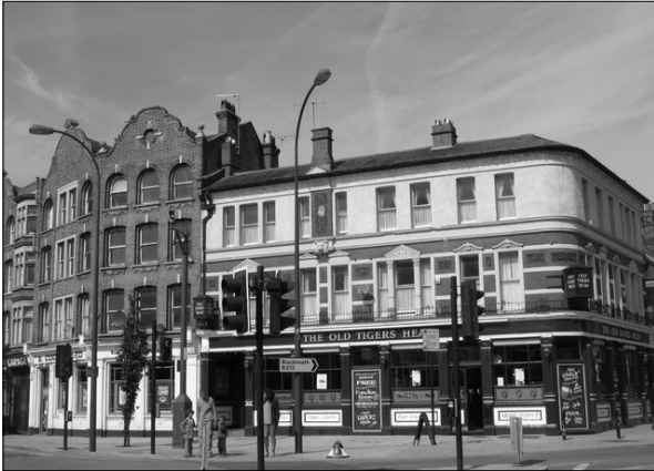
Figure 29 View of the pub from across the street
