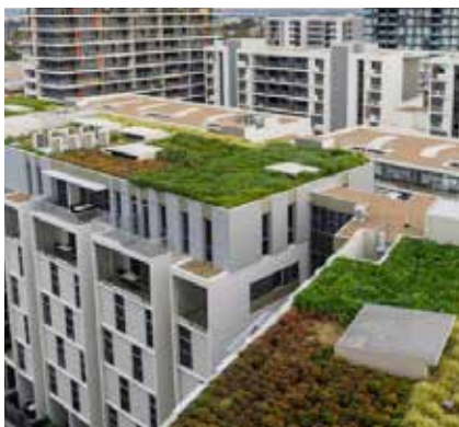
Figure 73: Urban green roofs.
