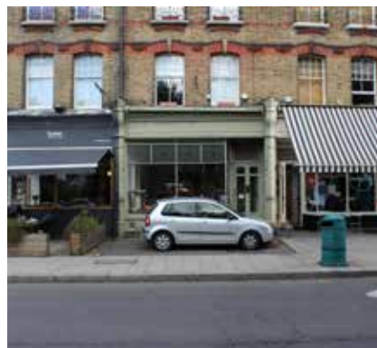
Figure 2: Shopfronts along Lee Road.
