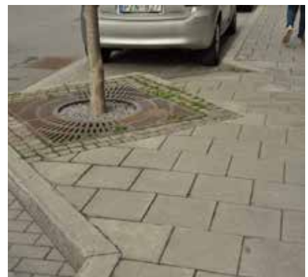
Figure 77: Drainage system around trees.
