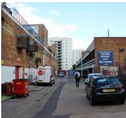
Figure 19: Poor quality streetscape and public realm.
