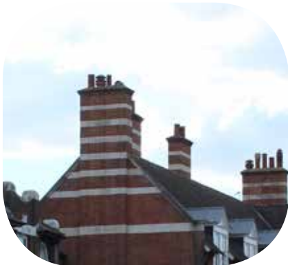
Figure 38: Combined red brick and white rendering on chimney.
