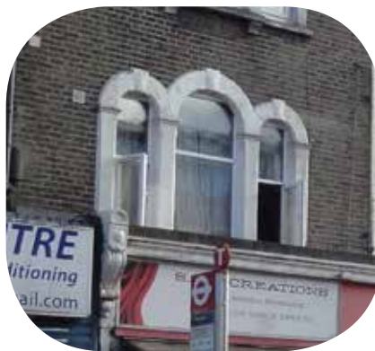
Figure 31: Masonry arches on triple window.
