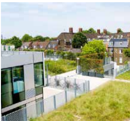
Figure 75: Urban green roofs.
