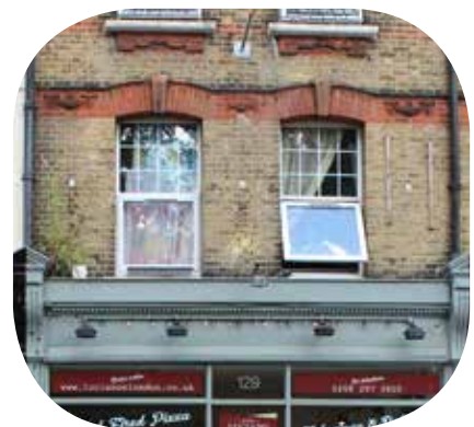
Figure 36: Red brick masonry details on windows.
