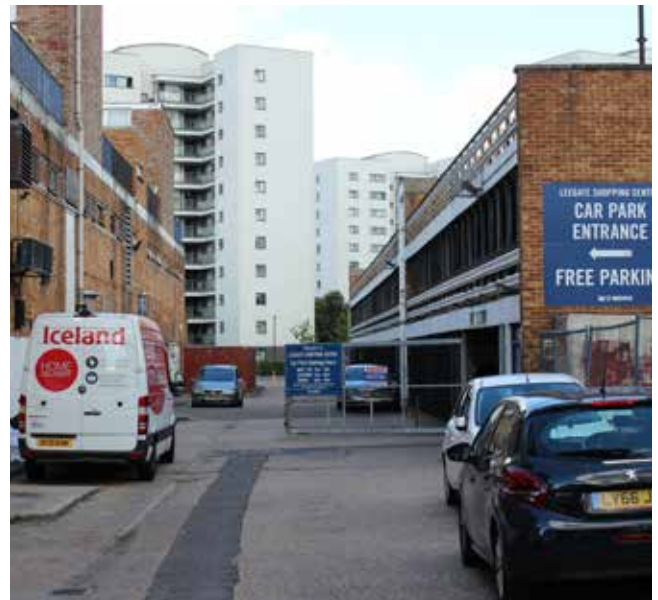
Figure 27: Underutilised sites and poorly laid out parking.
