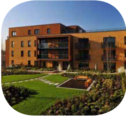
Figure 59: Mid-density apartment blocks with quality landscaping.
