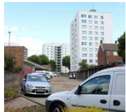
Figure 3: 10 storey towers, Leybridge Estate.
