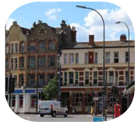
Figure 35: Continuous building line with various architectural detailing.
