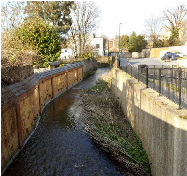
Figure 26: Visual obstruction of natural features.
