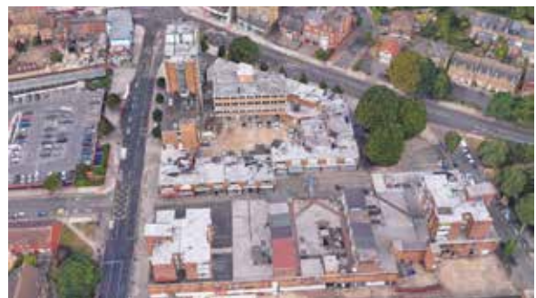
Figure 85: Leegate Centre (Site 4)
