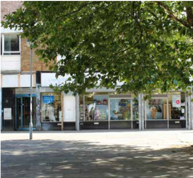
Figure 24: Vacant shops and poor quality shopfronts.
