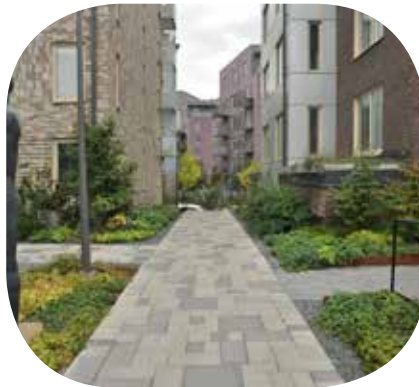
Figure 66: Secondary building façades facing into footways.
