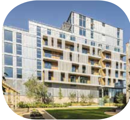
Figure 60: High-density apartment blocks with quality landscaping.
