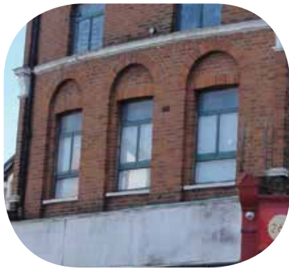
Figure 29: Masonry arches on windows.
