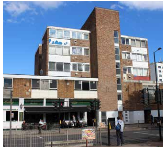
Figure 23: Low quality built environment.
