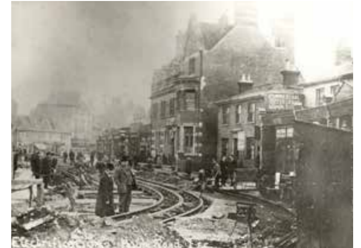
Tram tracks being laid on Lee High Road (c. 1907)
